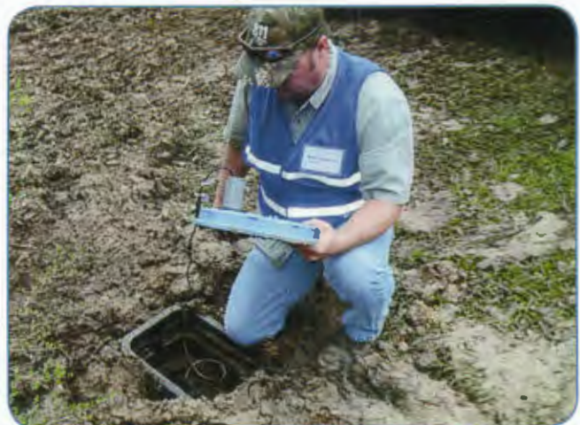
Michael Guimbellot, distribution, installs an ORION Cellular endpoint as part of the BEACON AMA managed solution.
